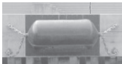
A fixed fender with double chain attachments
