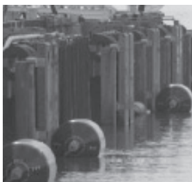
A floating fender with sliding sleeve and chain attachments.
